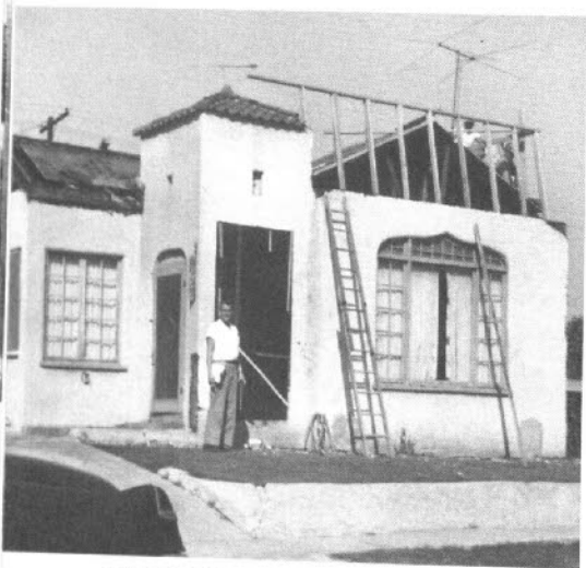
8937 Ashcroft Avenue in West Hollywood, remodeled by Larry Limotti and Ross Worsley in 1961-62. The framing for the mansard roof goes up on the 1920s bungalow. Photo by Larry Limotti.
