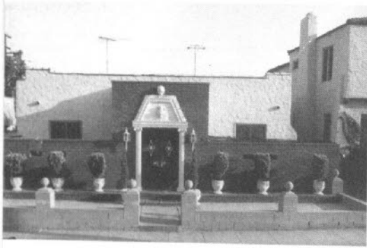
8834 Rangely Avenue, West Hollywood. Benjamin and Betty Heiman's 1968 remodel of their house. Designed by Benjamin Heiman. This facade was removed in 1999.
